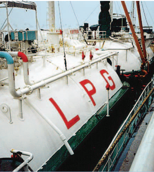
Odorization of LPG (Liquefied Petroleum Gas) during ship loading
